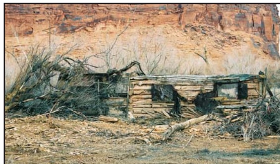
Log cabin located on Moab site prior to demolition.
