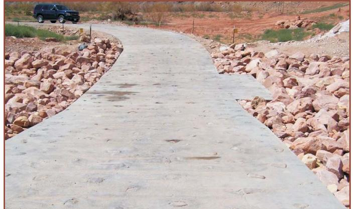
*The lower Moab Wash crossing was completed in May. A rock apron abuts each side of the grouted rock crossing.*
