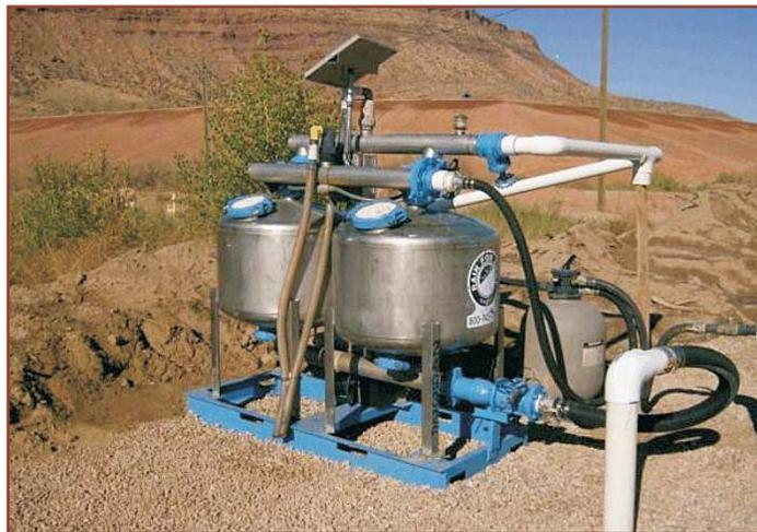
This filtration system (now enclosed) removes silt and sediment from the pond water before it is injected into the infiltration trench.
